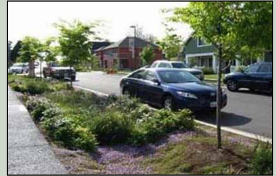
Vegetated swales slow, infiltrate, and filter stormwater runoff. They are well suited along streets and parking lots. (Source: http://www.3riverswetweather.org/green/green-solution-vegetated-swale )
